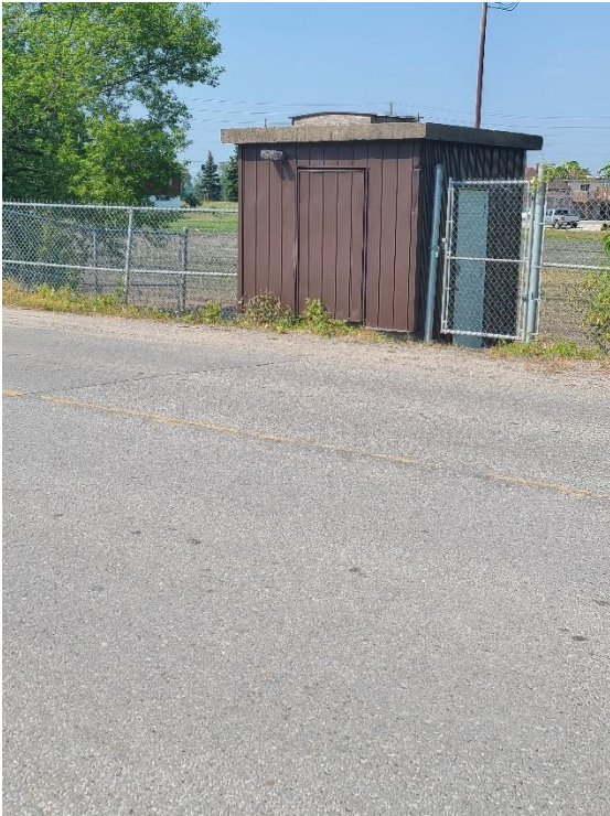
Figure 1 Proximity to Canal Road
